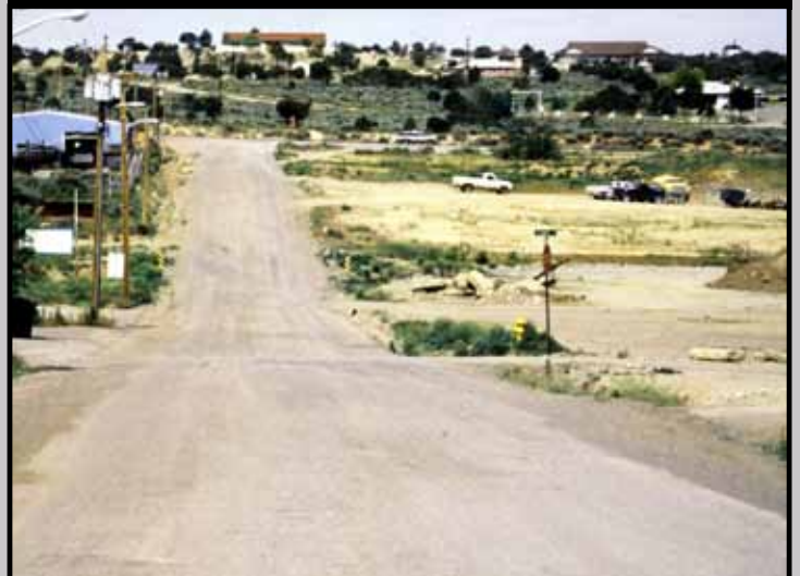
Aggregate Stabilized with EMC SQUARED® Stabilizer (utilized for two years as a street surface)
