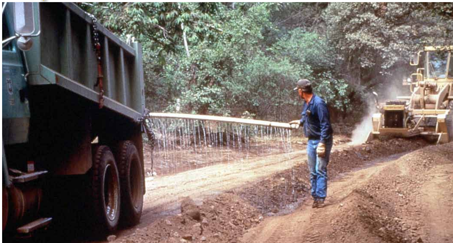
EMC SQUARED® Stabilizer application
