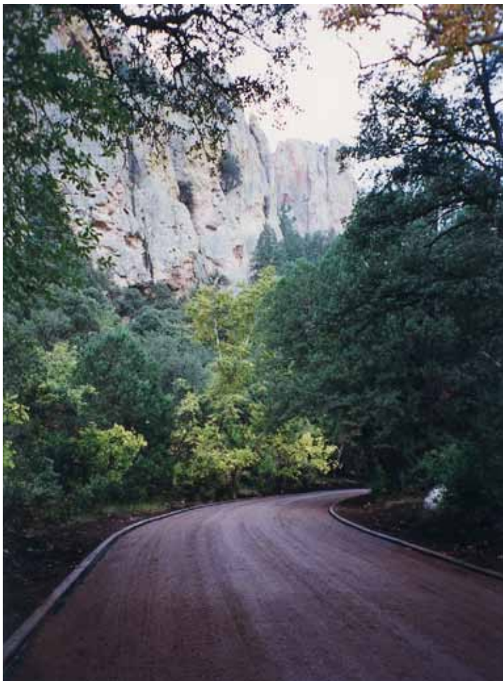
Road prepared for paving
