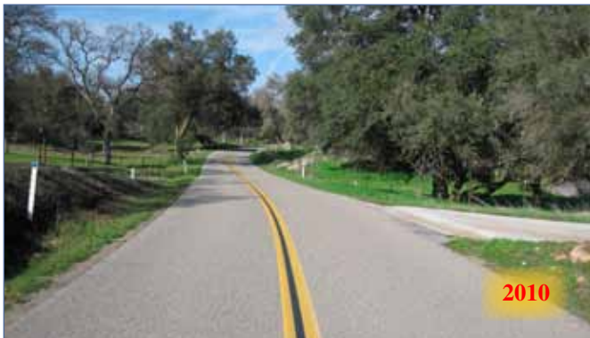
Asphalt pavement surface above stabilized base in excellent condition after thirteen years of service.
