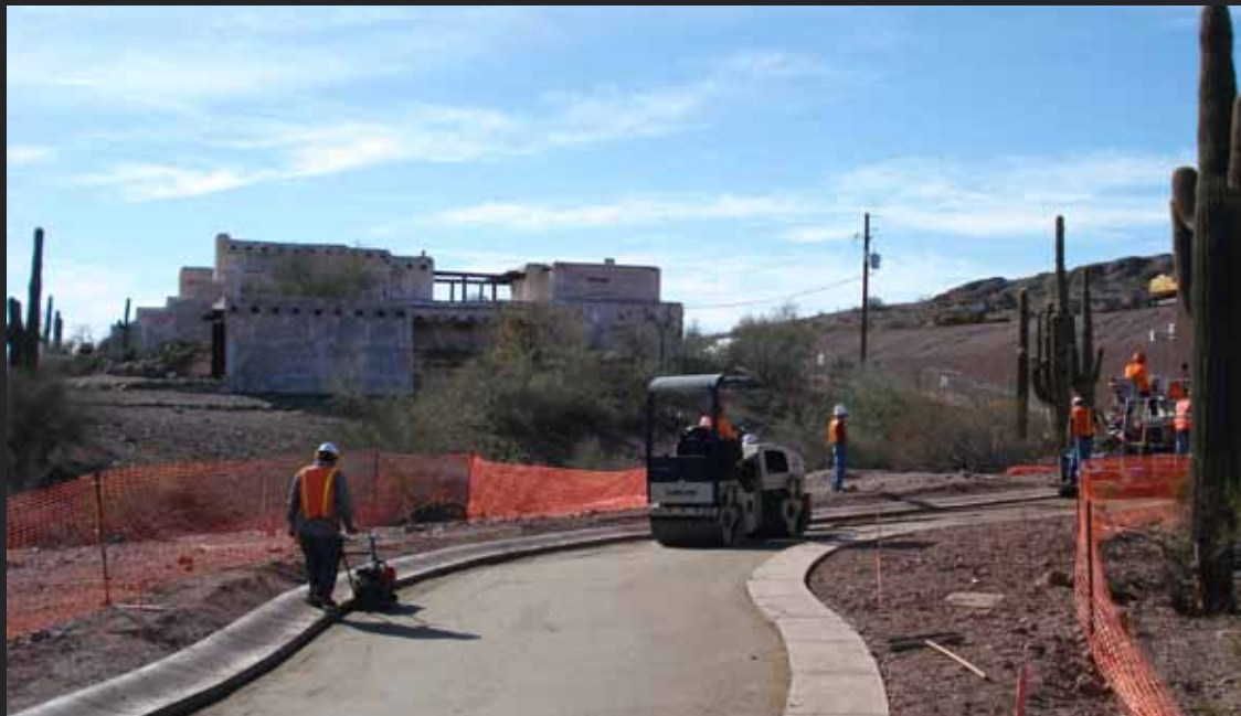
Final Compaction
