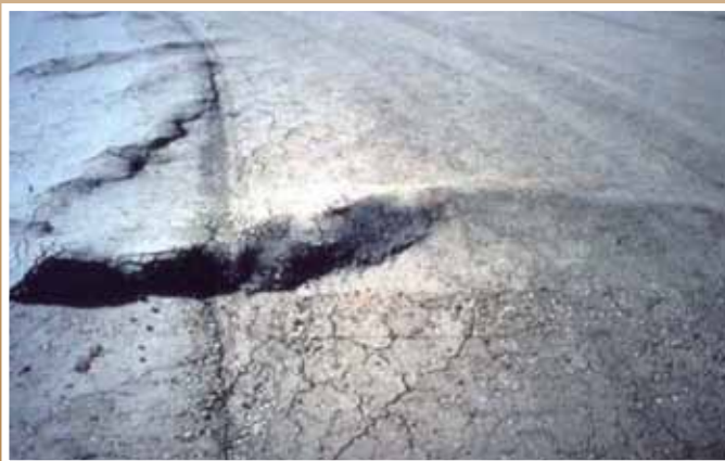
EXAMPLES OF SULFATE-INDUCED DAMAGE
