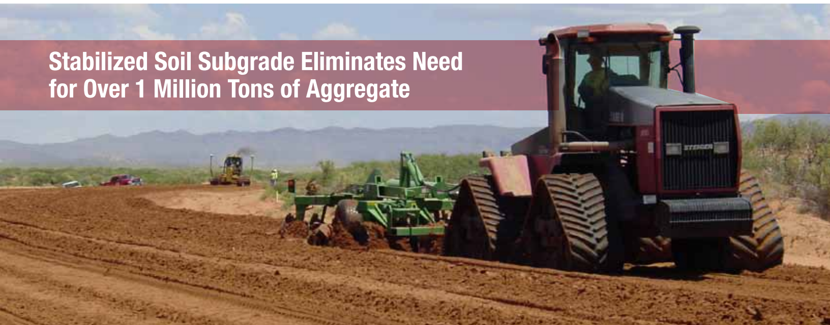
Subgrade Stabilization with Disc Mixing of EMC SQUARED Stabilizer Treatment
