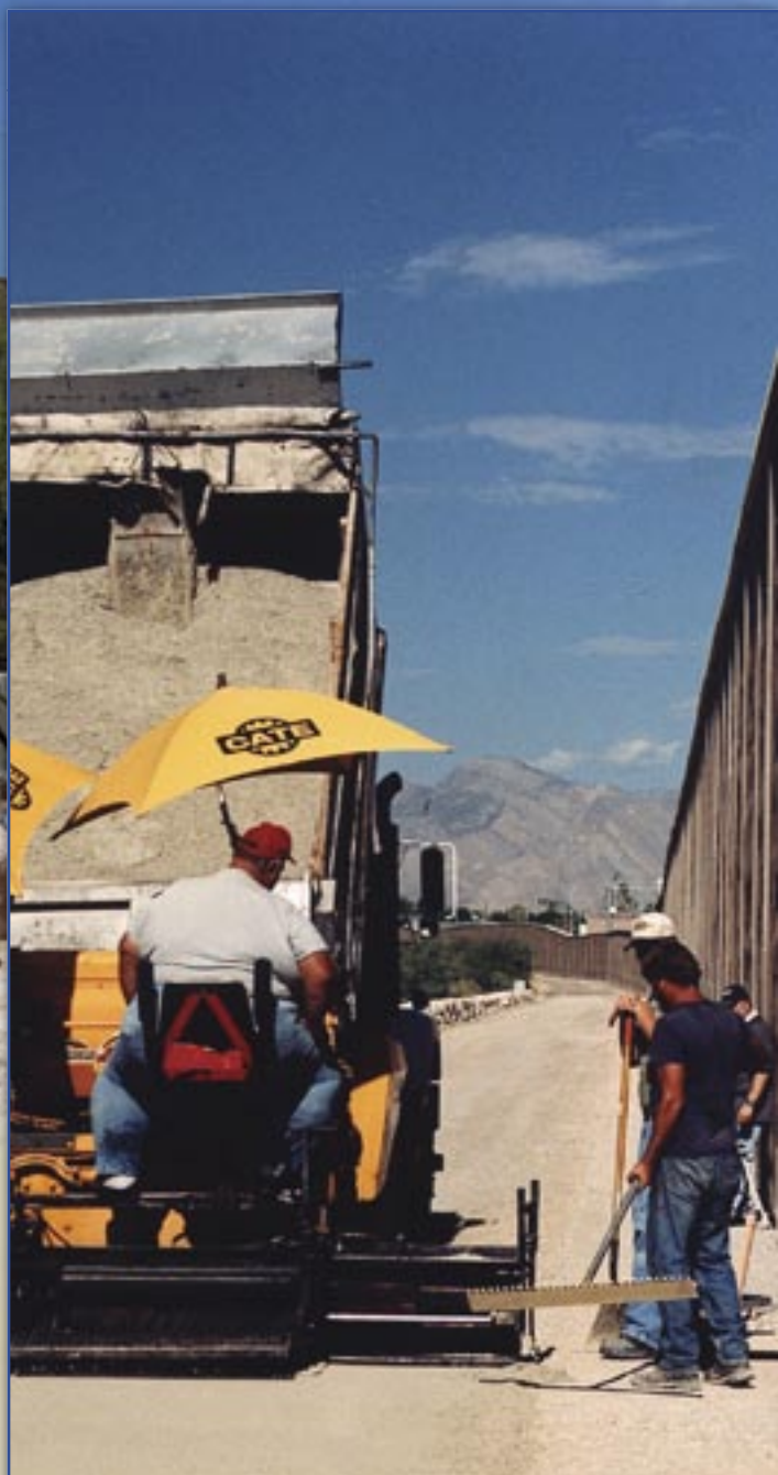
Paving In Progress On Stabilized Base
